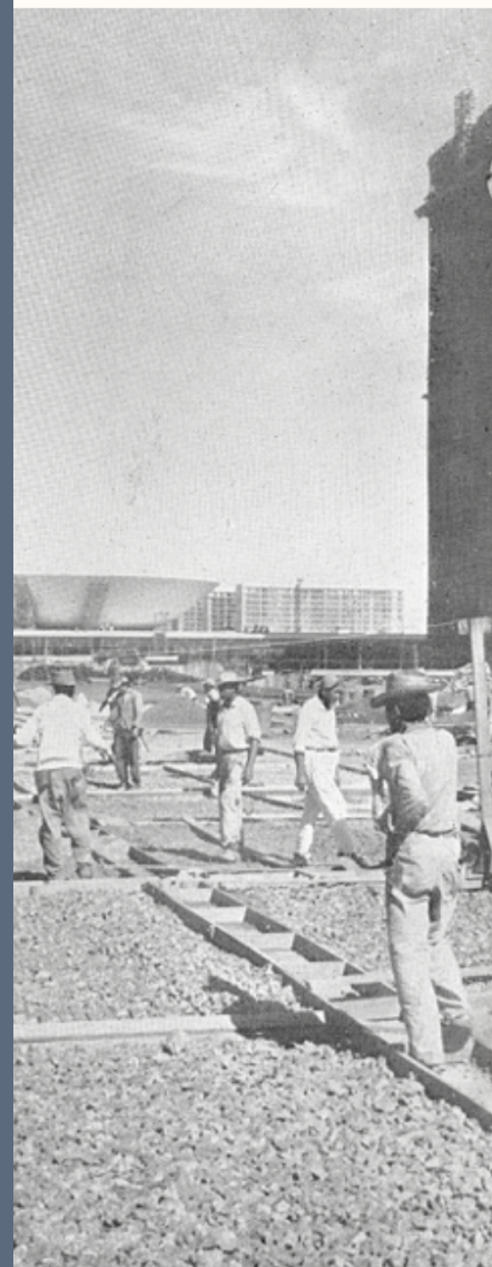
Construction of the National Congress
