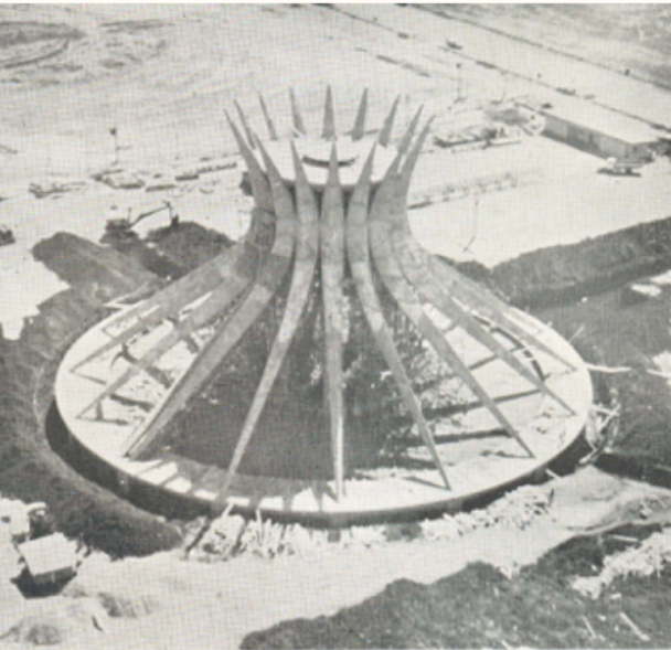
Construction of the Cathedral of Brasília
